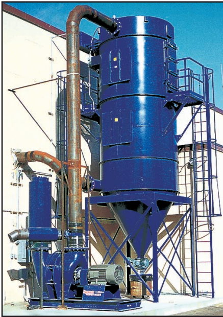
Power Mizer vacuum producer with pulse-type separator providing a continuous duty, high velocity dust collection system at a printed circuit board manufacturer.
